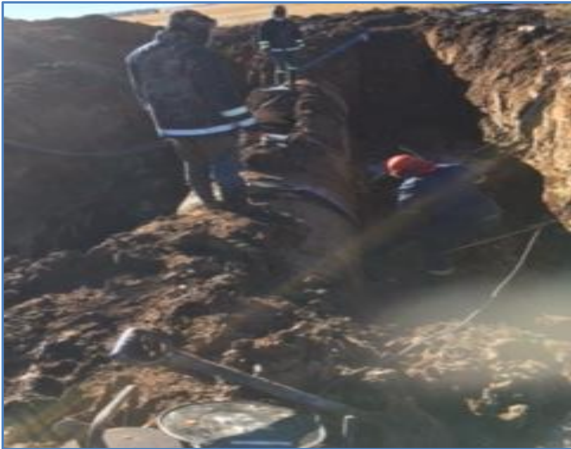
Maintenance team at work
