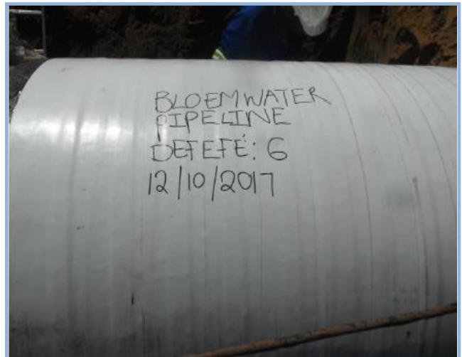
Cathodic protection before installation
