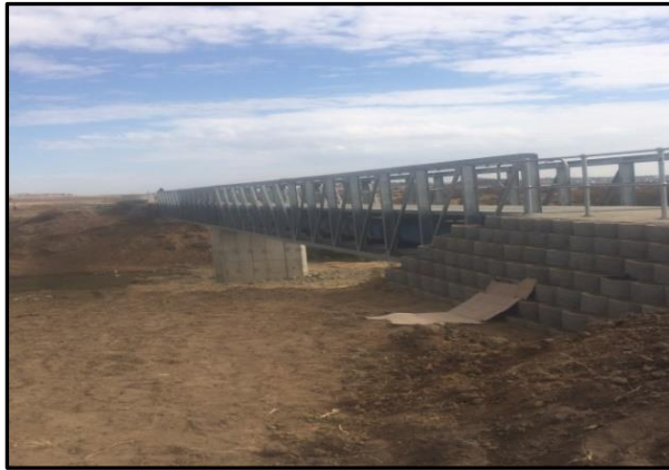
Steel bridge for pedestrian and pipeline
