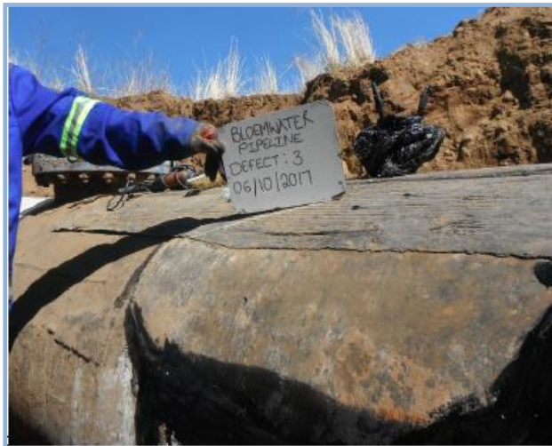
Cathodic protection before installation
